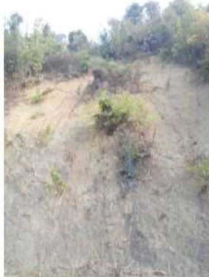
Landslide location code: L-5
