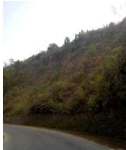
Landslide location code:L-15
