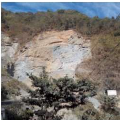
Landslide location code: L-2
